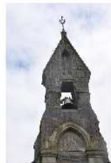
490(2) - 10,top of the frontal tower
