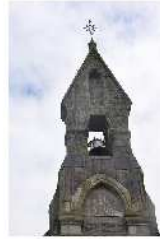
498(2) - 10,top of the frontal tower
